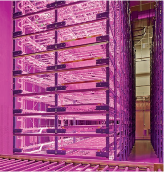
Higher environmental temperature uniformity is achieved with LED lights, at a much lower energy input. Lights are also low voltage and waterproof.
