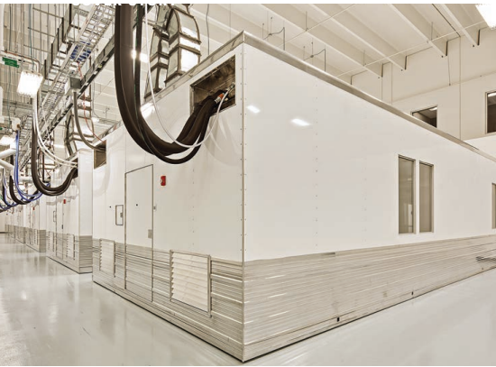
Each G-CON POD is served by its own independently controlled, redundant HVAC system.
